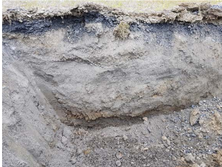
Plate 7.2 – Typical subsurface profile as encountered in TP3
